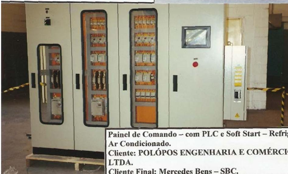
**Painel de Comando – com PLC e Soft Start – Refrig.**
